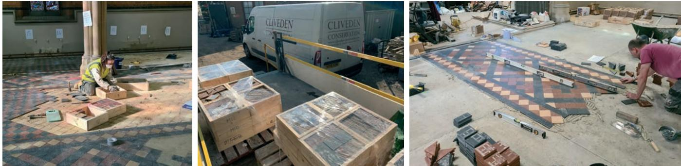
➡ **THE VICTORIAN TILED FLOOR** at All Saints Church in Boyne Hill, Maidenhead – designed by G E Street in 1857 – had become deteriorated and unsafe due to being laid on a defective substrate. Quantity surveyors Sawyer and Fisher and architect Roderick Maclellan recommended well-known specialists Cliveden Conservation to carry out the sensitive repair of the floor in accordance with Street's original design.
